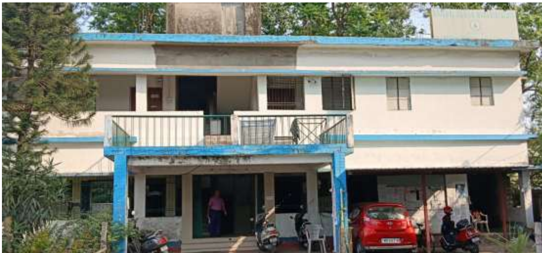
Well maintained parking place in front of administrative building
