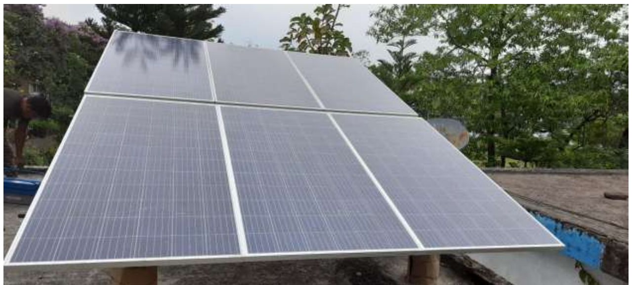
Installation of Solar PV cell
